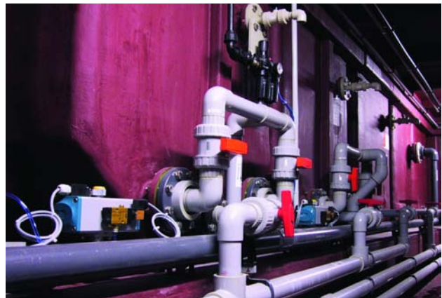
Picture 6: Dry cellar: no aggressive fumes attack the sensitive equipment
