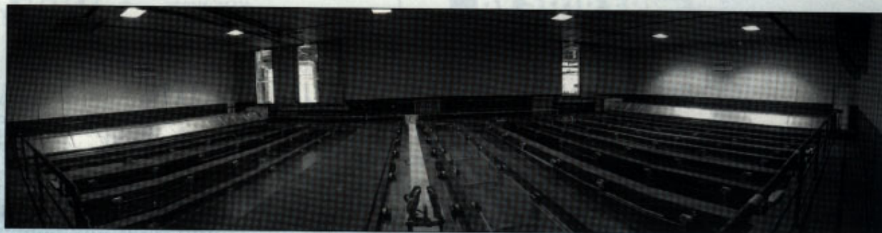
Figure 2. Encapsulated pickling area
